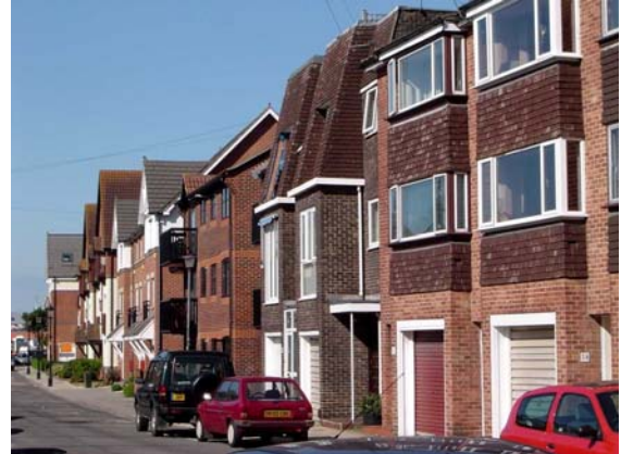
Most of the 1970s and 1980s developments on Warblington Street have allowed cars to dictate the design
